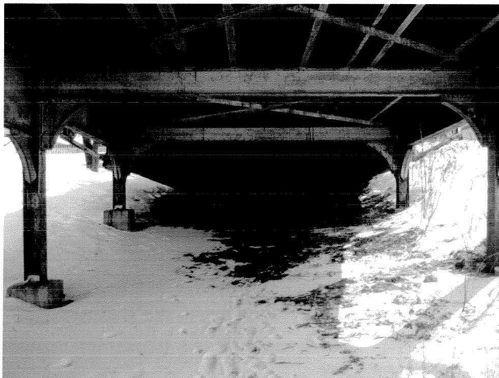
Photo 02: South Abutment and Bent-Piers
