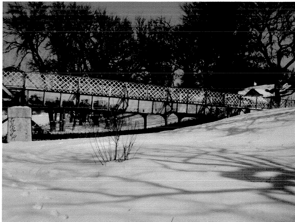
Photo 01: South End of the Existing Bridge, Looking East
